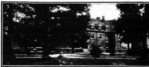
FRONT VIEW, MAIN BUILDING
